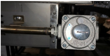
Step 3: LP gas "Hard Plumed" conversion. Unscrew regulator cap.
